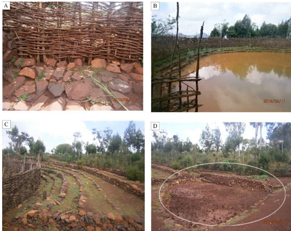
Figure 1:(a) A wooden mesh to sieve debris,(b) fenced pond, (c) preserving ponds from silt by constructing outside terraces, and (d) basins to collect silt coming in through the flood (Behailu, Pietilä & Katko 2016)
