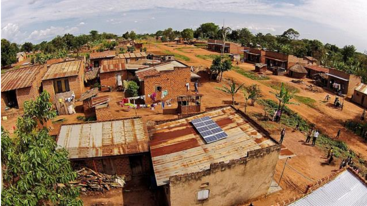
Figure 5 The 500 W solar system powers a home, a public broadcasting system, a barbershop and a video hall in a rural village in Uganda.
